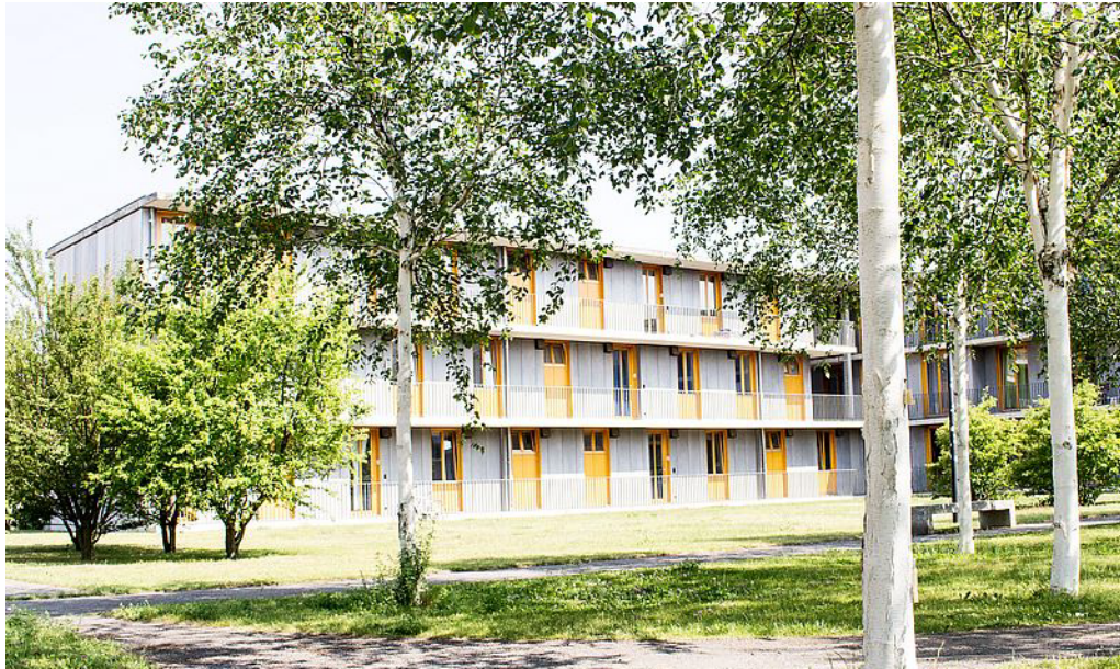
Student residence hall at Zanderstraße 10
